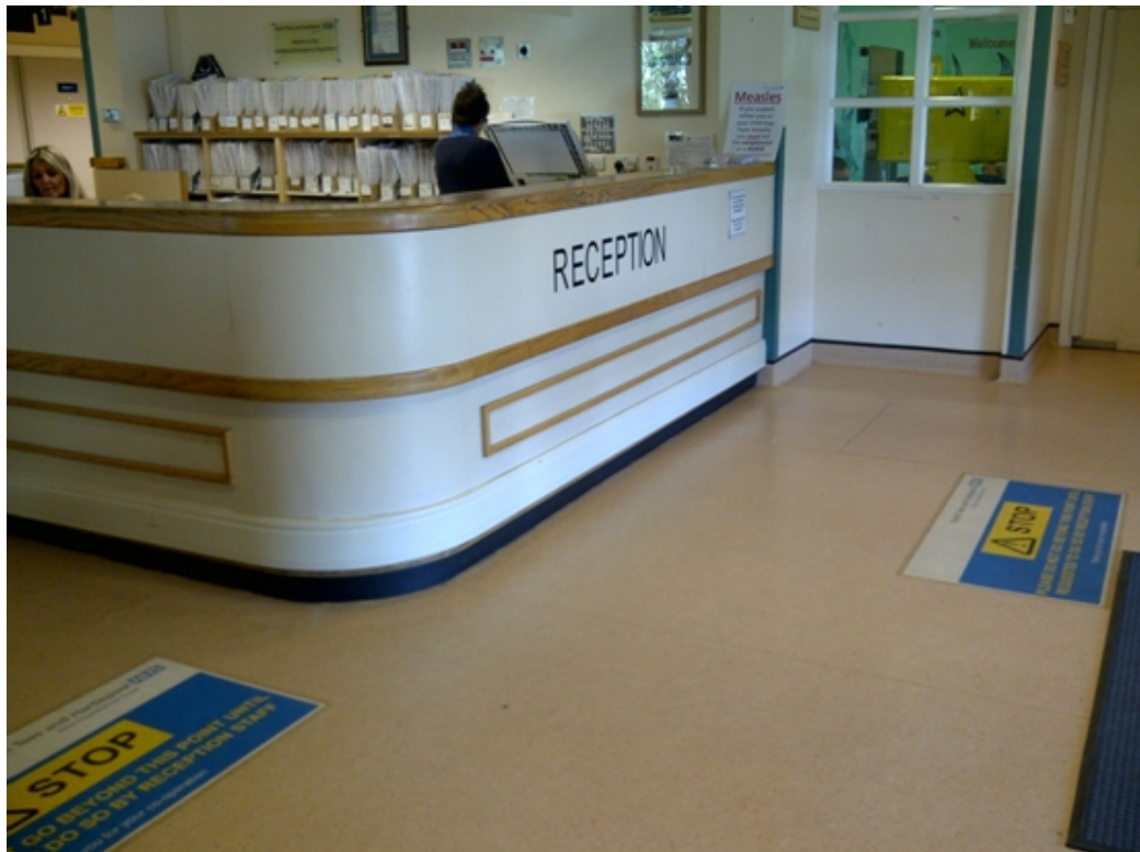
ThermaSkirt provides the heating and skirting in one – here seen curved around the reception desk.
